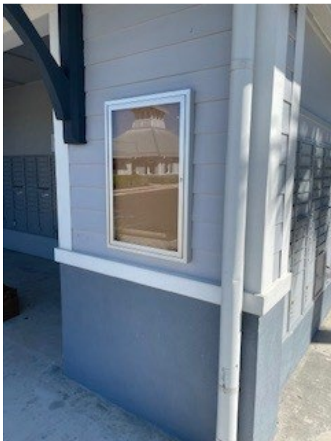
New bulletin board installed.
