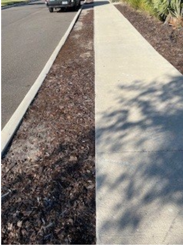
Front sidewalk work to start week of 11/17.
