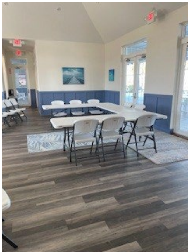
Clubhouse painting in progress.
