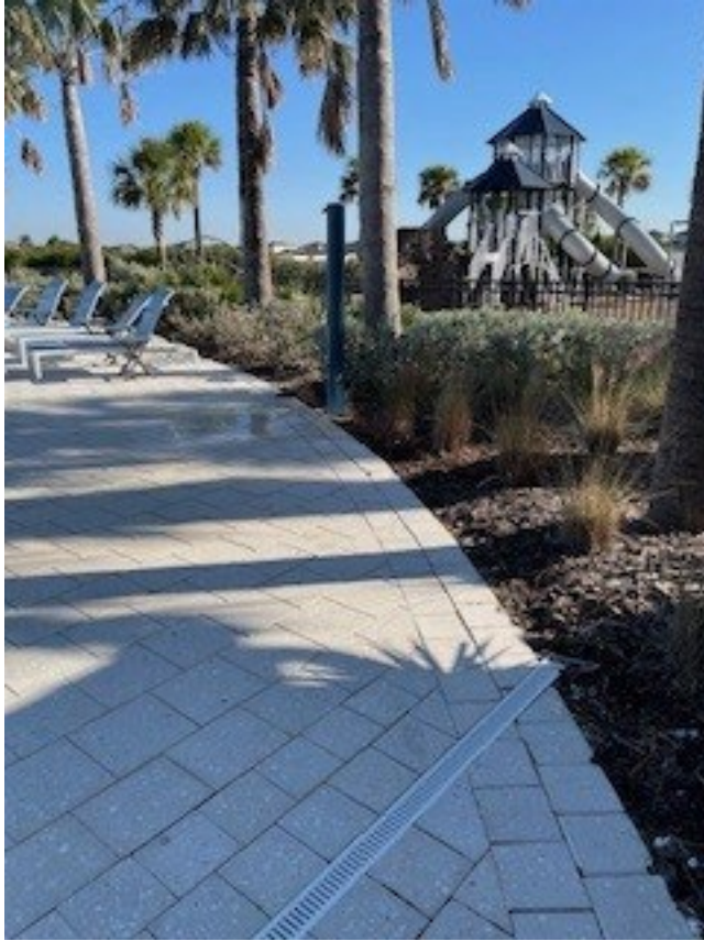
Shower to pool repaired 11/14.
