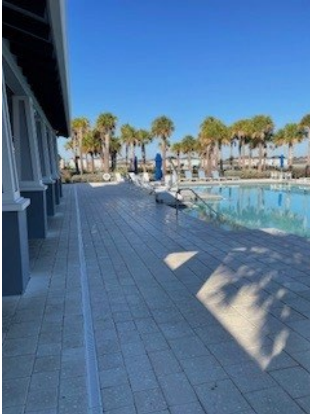
Pool area looks good palms need trimming.
