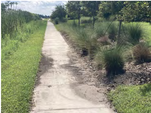
Sidewalk On 11th Street 1
